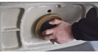
9.Turn over the toilet bowl and install the flange ring as below picture
