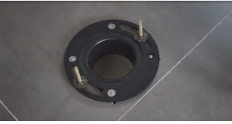
6.Install two long screws as below picture
