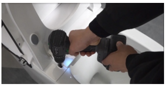
7.Unscrew the screws on the toilet seat
