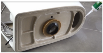
10.Apply some glass glue on the bottom of the toilet (The glass adhesive in the picture needs to be purchased by oneself.)
