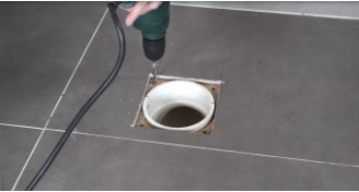
3.Take off the flange ring and drill four holes for screws
