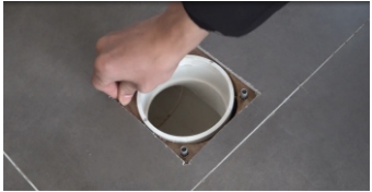
4.Put the screws into the holes
