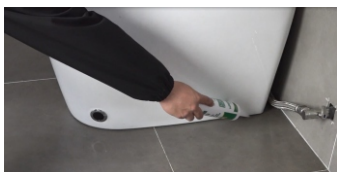
15.Apply some glass glue to fix the toilet and insulate the outside dirt from entering.(The glass adhesive in the picture needs to be purchased by oneself.)
